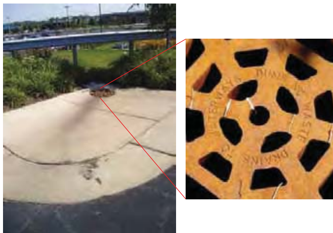
Runoff from sealcoated pavement (black surface) enters storm drains that lead to local streams. Drain grate (inset) is marked “DUMP NO WASTE” and “DRAINS TO WATERWAYS.”
