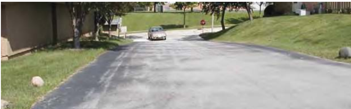
Gray asphalt pavement shows through where sealcoat has worn off the driveway of an apartment complex.
