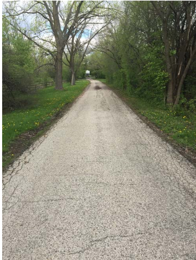
Fig.16 - Tamarack Lane intersection facing north
