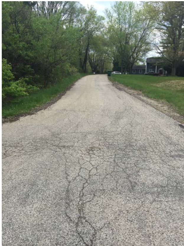
Fig.15 - Tamarack Lane intersection facing south
