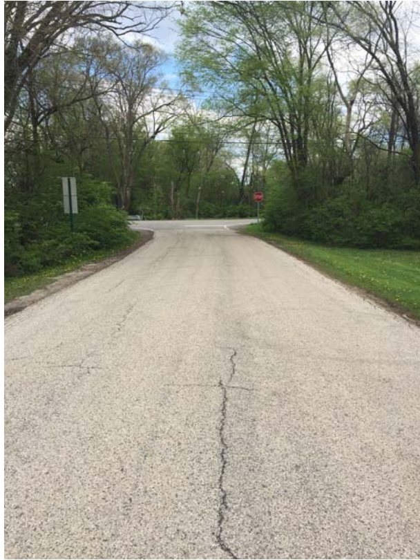
Fig. 10 - Woodcreek Road facing north towards intersection with IL-68 (Dundee Road)
