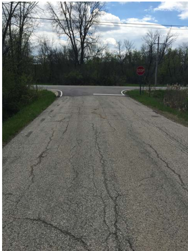
Fig. 21 – Facing south toward intersection of Lakeview Lane and IL-68 (Dundee Road)
