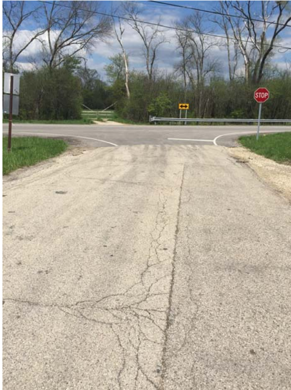
Fig. 6 - Healy Road facing north toward intersection with IL-68 (Dundee Road)
