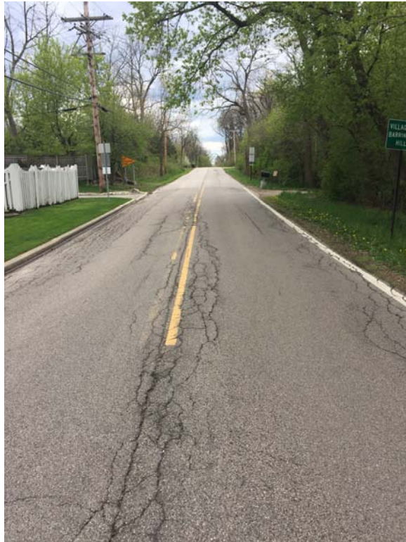
Fig. 4- Helm Road from village limits facing east
