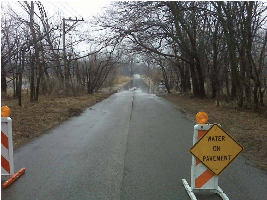
March 2009 Flooding Condition on Chapel Road
