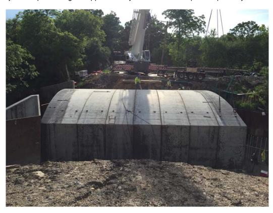
Major work items remaining include construction of the north wingwalls, placement of backfill, and reconstruction of the concrete bridge deck and approach pavements. As a reminder, there will be periods of time in which the Buckley/Cuba intersection will need to be closed to facilitate drainage and pavement improvements.
