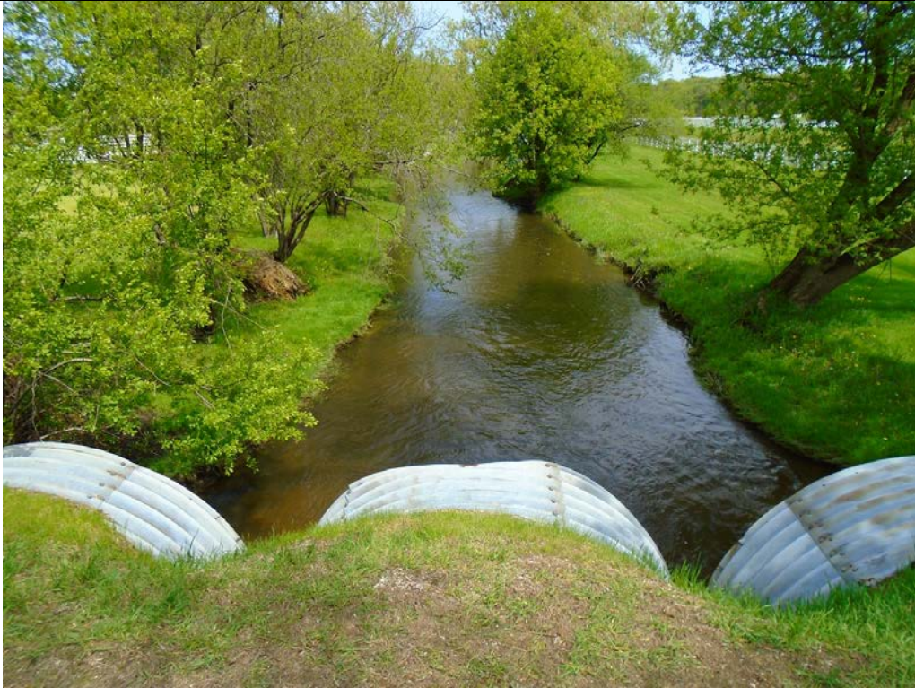
2) LOOKING AT NORTH CHANNEL
