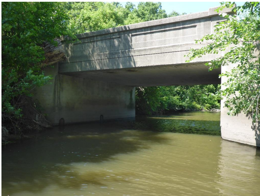
Figure 2. Bridge elevation looking northwest.
