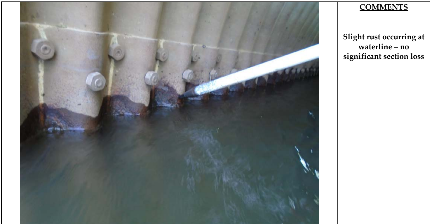
6) VIEWING RUST AT WATERLINE
