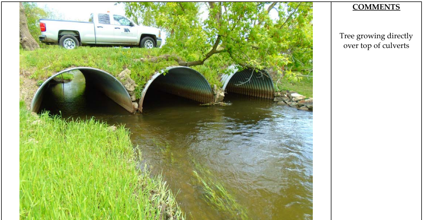
4) LOOKING AT SOUTH END OF CULVERTS
