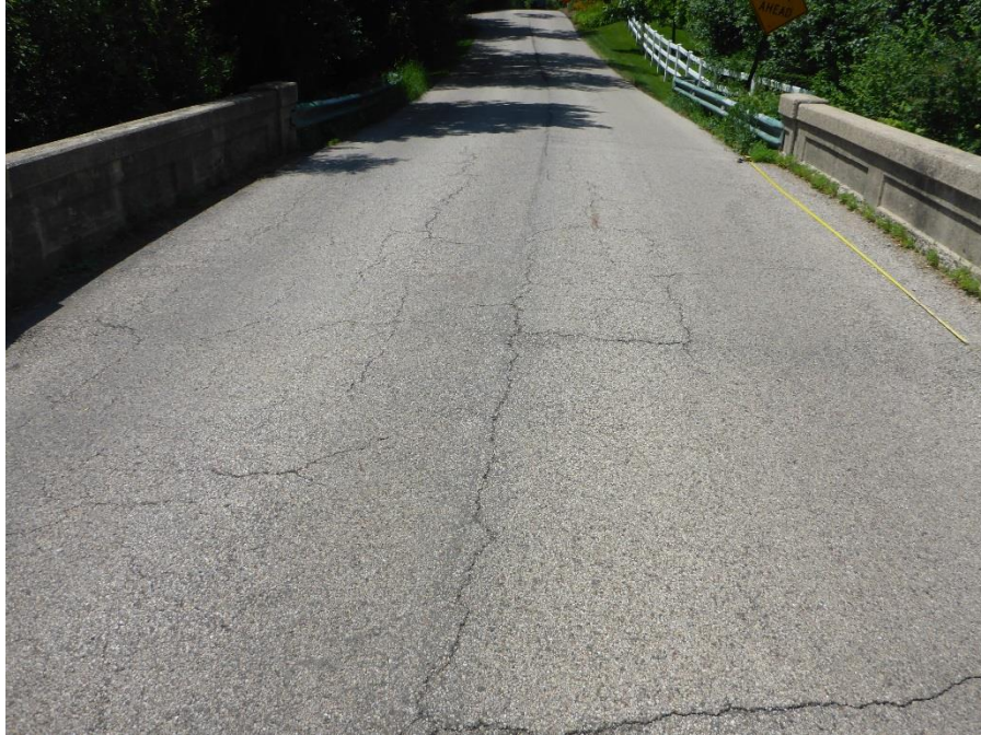
Figure 1. Porter Bridge looking west.
