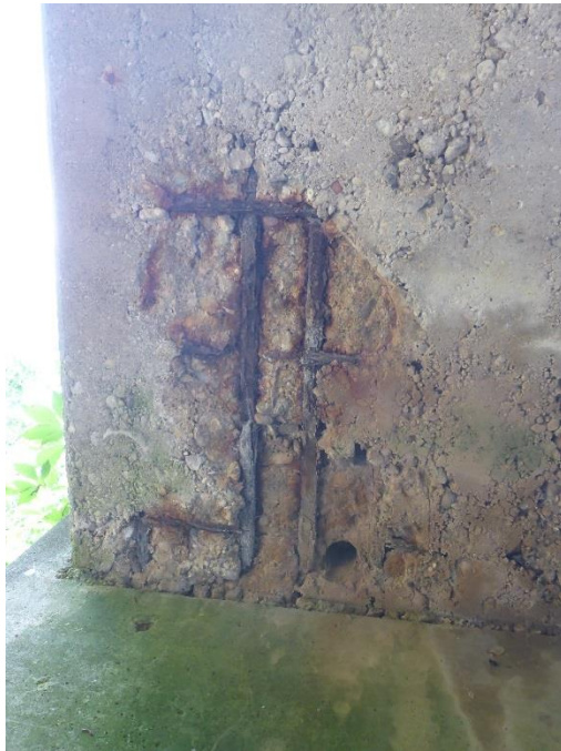
Figure 3. Spalled concrete and exposed reinforcing bars at northeast corner of deck soffit with water staining.
