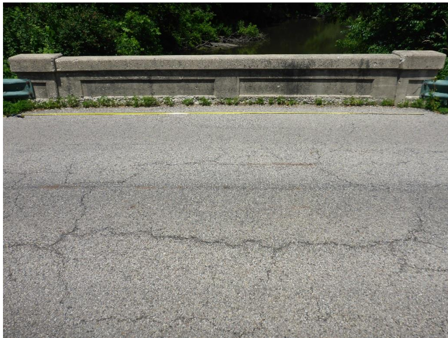
Figure 4. North parapet with freeze/thaw deterioration and vegetation along base.
