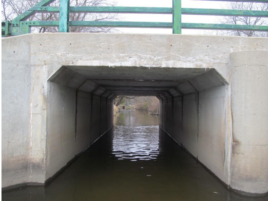
Figure 3. Typical view of the culvert interior.
