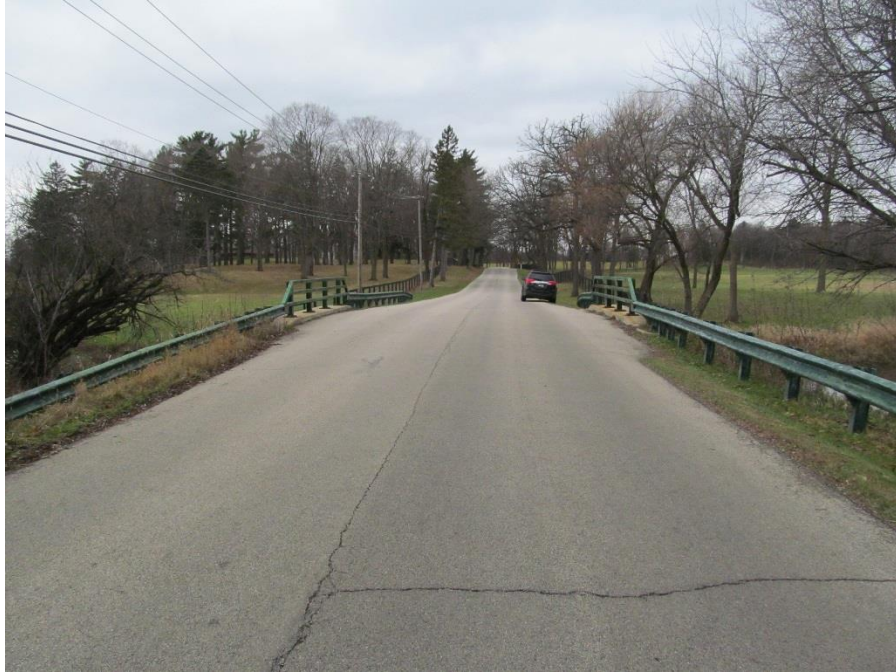
Figure 1. Green Rail Bridge looking northwest.
