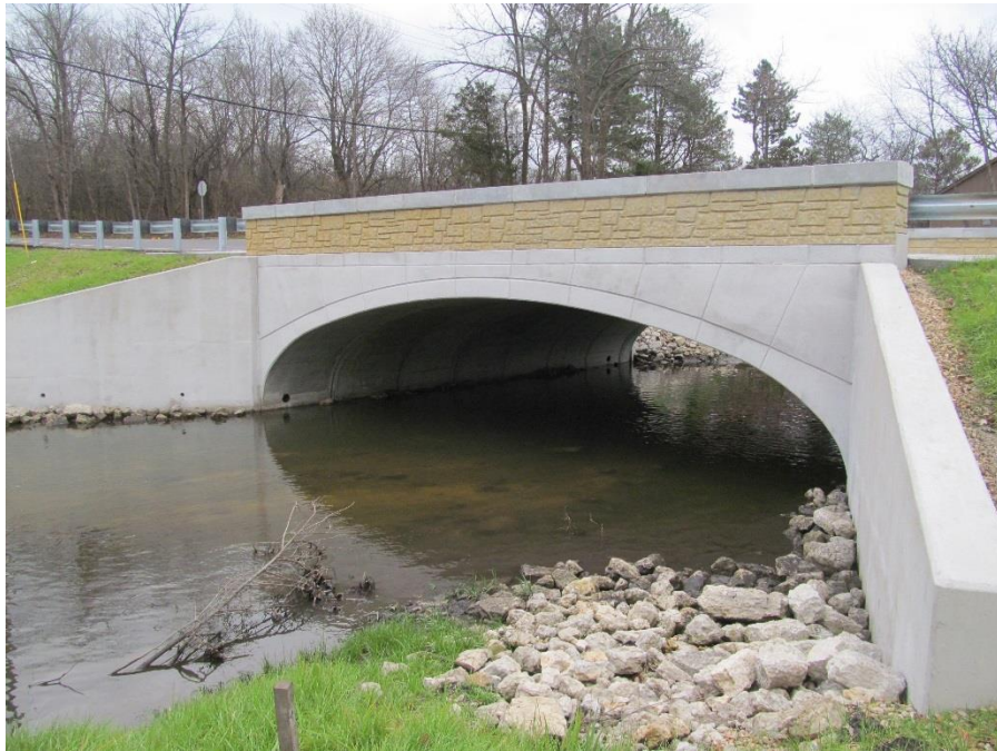
Figure 1. West Cuba Road Bridge looking southeast.
