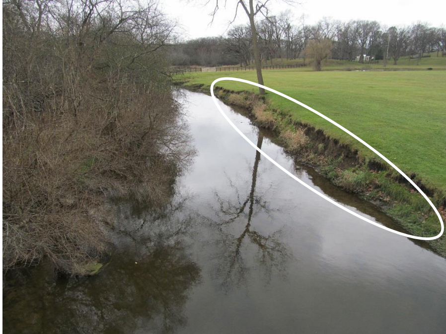
Figure 11. View of the channel facing southwest, note circled area shows sloughing / erosion of the west channel bank.
