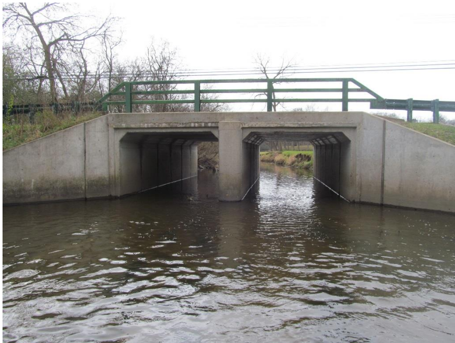
Figure 2. Elevation of the two-cell box culvert looking southwest.
