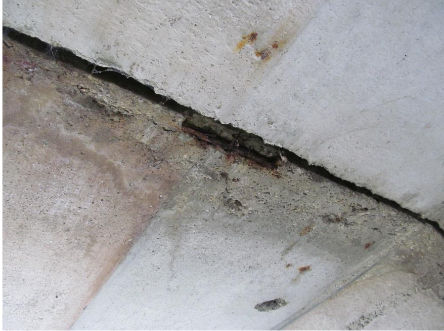
Figure 7. Unrepaired spall and exposed reinforcing steel in the concrete soffit.
