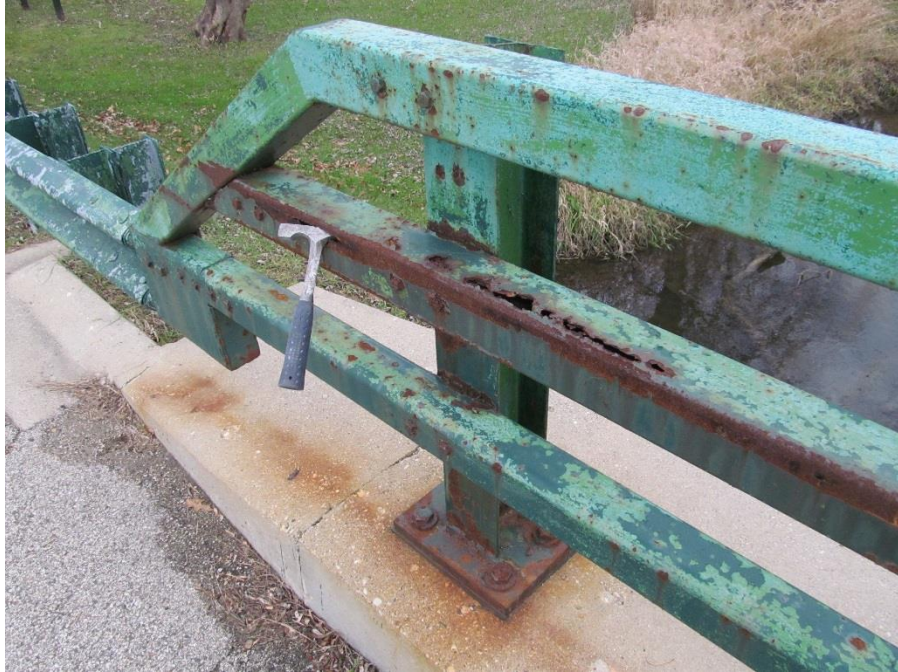
Figure 9. North steel bridge rail exhibiting corrosion with thru-thickness section loss in the middle rail.
