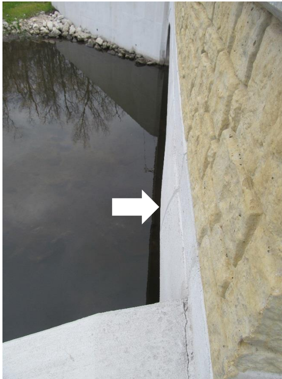
Figure 3. Bulge in north concrete headwall (arrow) at west abutment (looking east).
