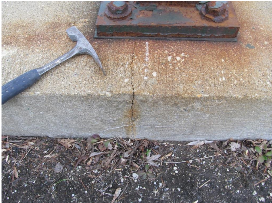
Figure 10. Cracking in culvert headwall, observed at isolated locations on both headwalls.
