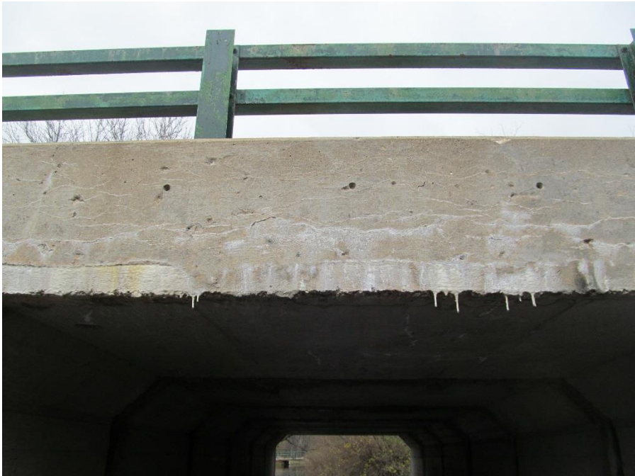
Figure 4. Freeze-thaw cracking and efflorescence observed at the concrete headwalls.
