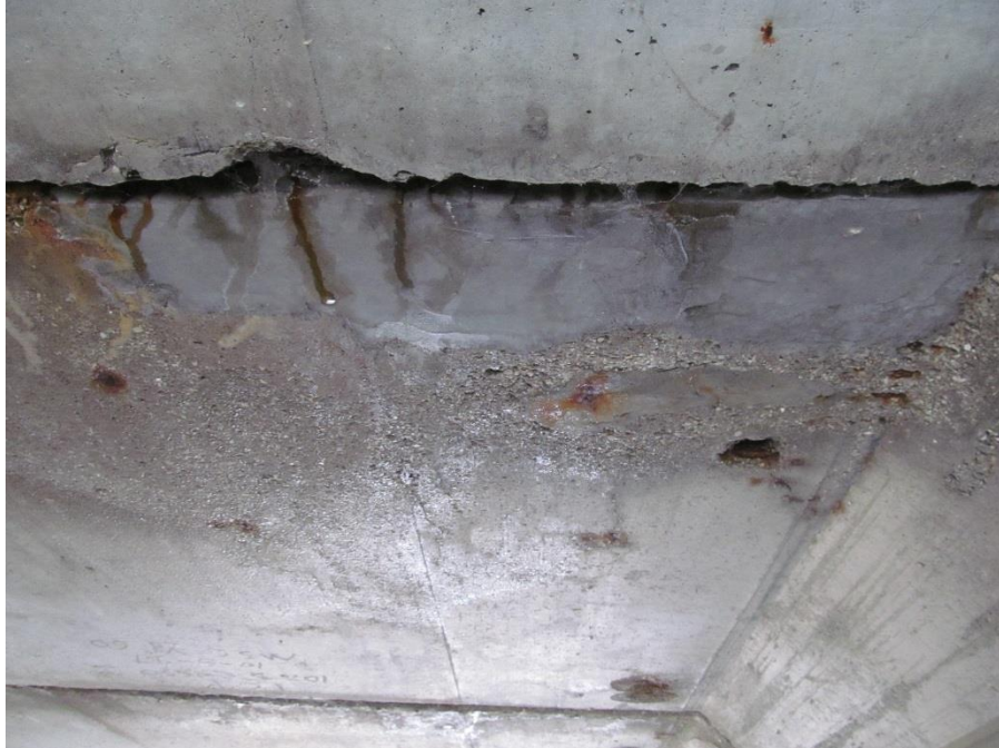
Figure 5. Area of repaired concrete on the soffit (east cell) showing indications of moisture staining through the joint.
