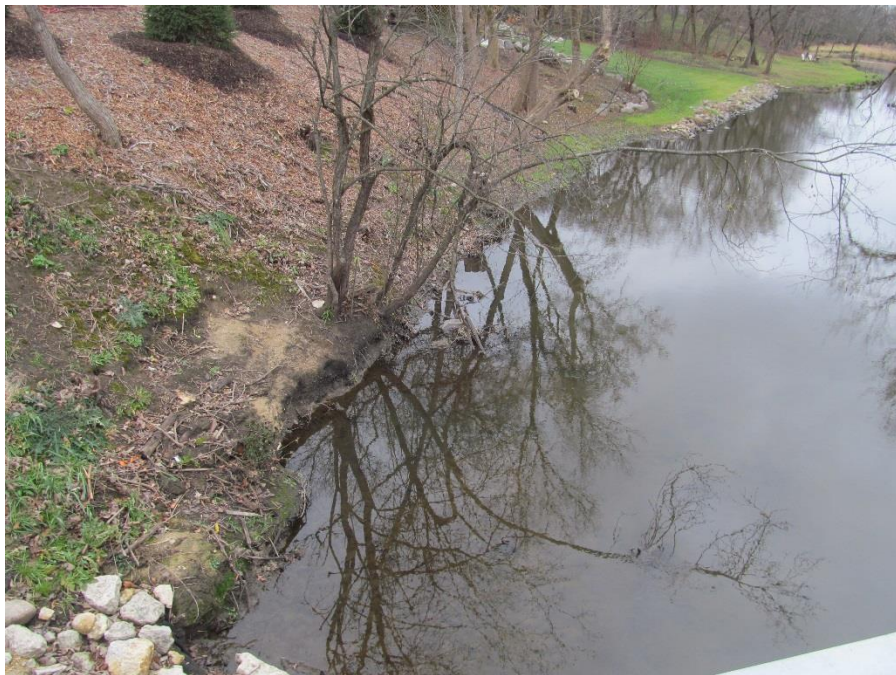
Figure 2. Lack of vegetation along east channel bank, (looking south).
