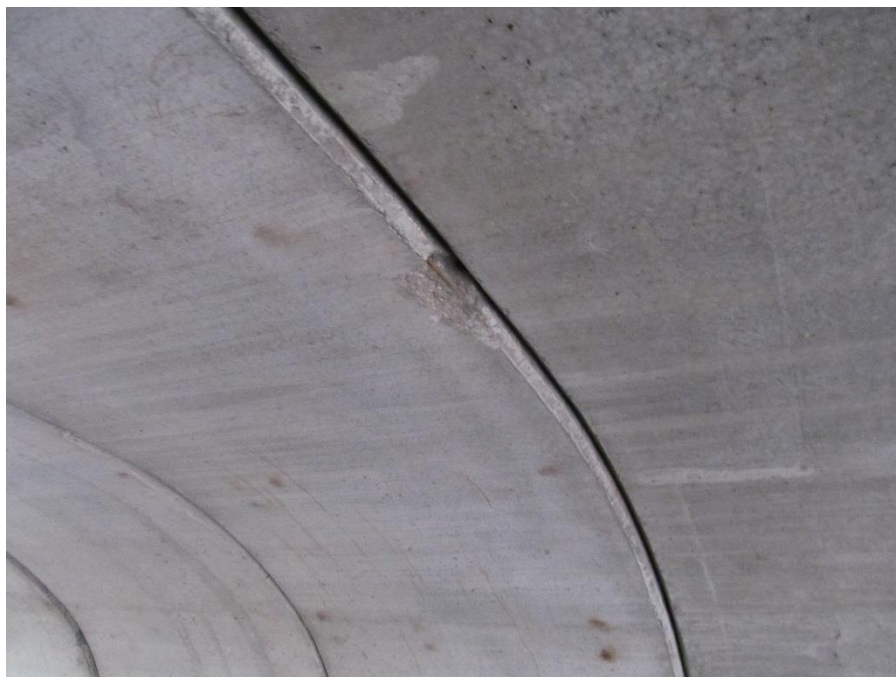
Figure 4. Spall in precast segment joint with exposed reinforcing steel.
