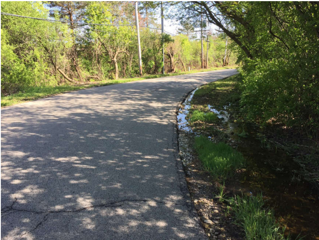
Fig. 11 – W. Cuba Road- Eroded Ditch Drainage
