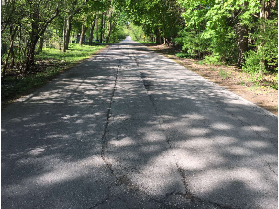
Fig. 5 – Old Hart Road facing north toward Oak Knoll Road
