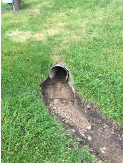
Downstream End- River Rd. Culvert
