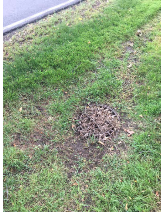
Upstream Inlet- River Rd. Culvert
