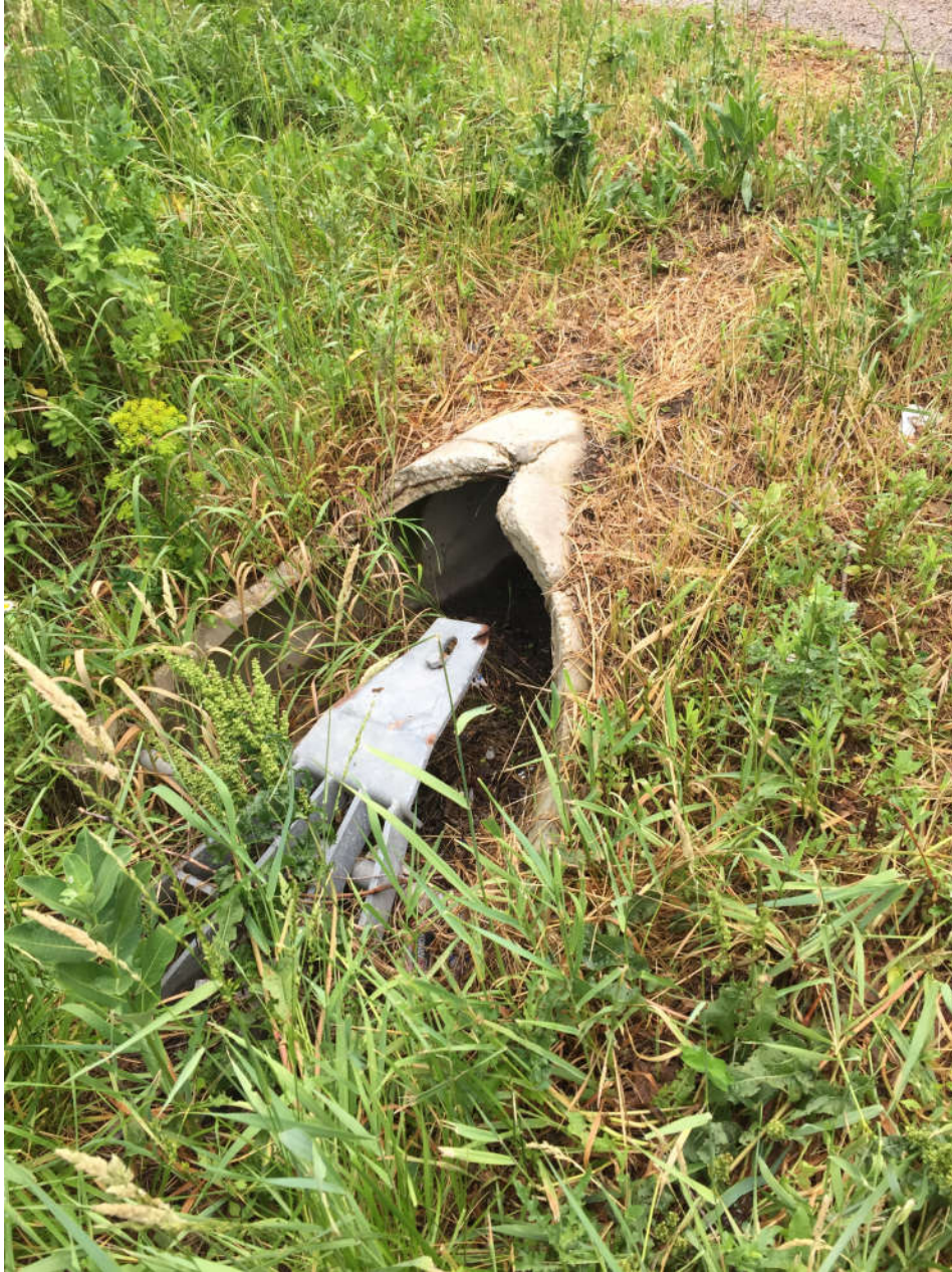
Damaged Flared End Section- Springwood Lane
