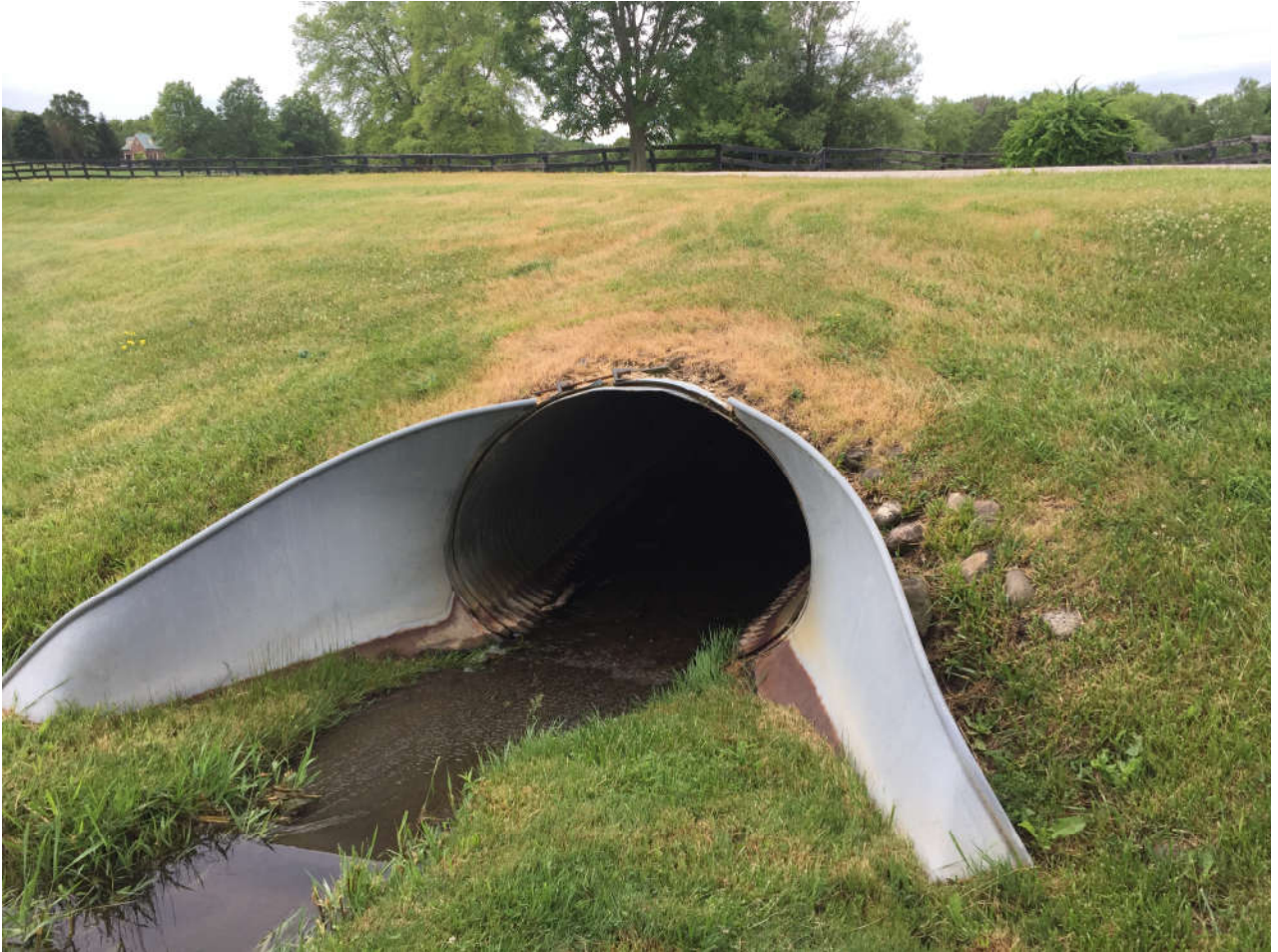
48"x63" Elliptical CMP @ 20 Creekside Lane
