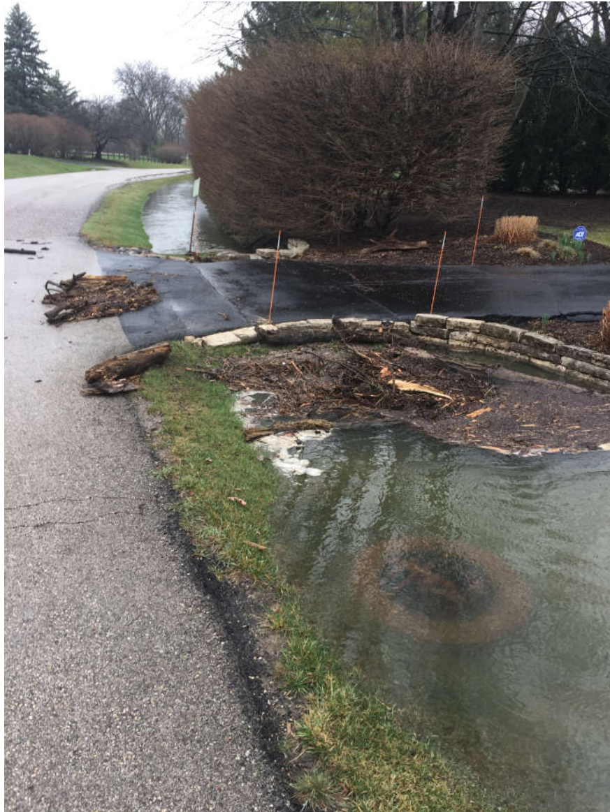
Three Lakes Road Ditch Inundation- April 2017
