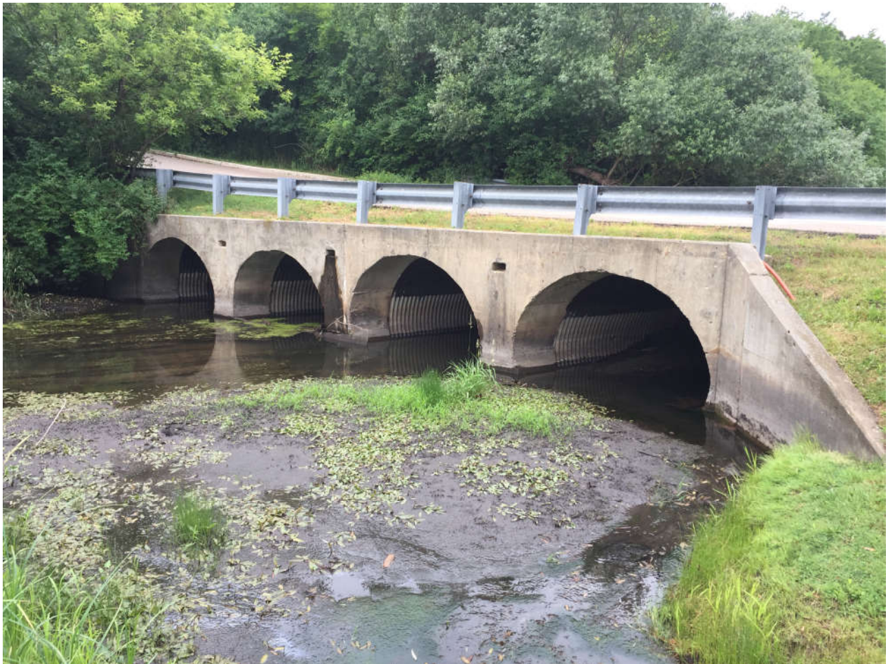
Spring Creek Crossing at Rock Ridge Road
