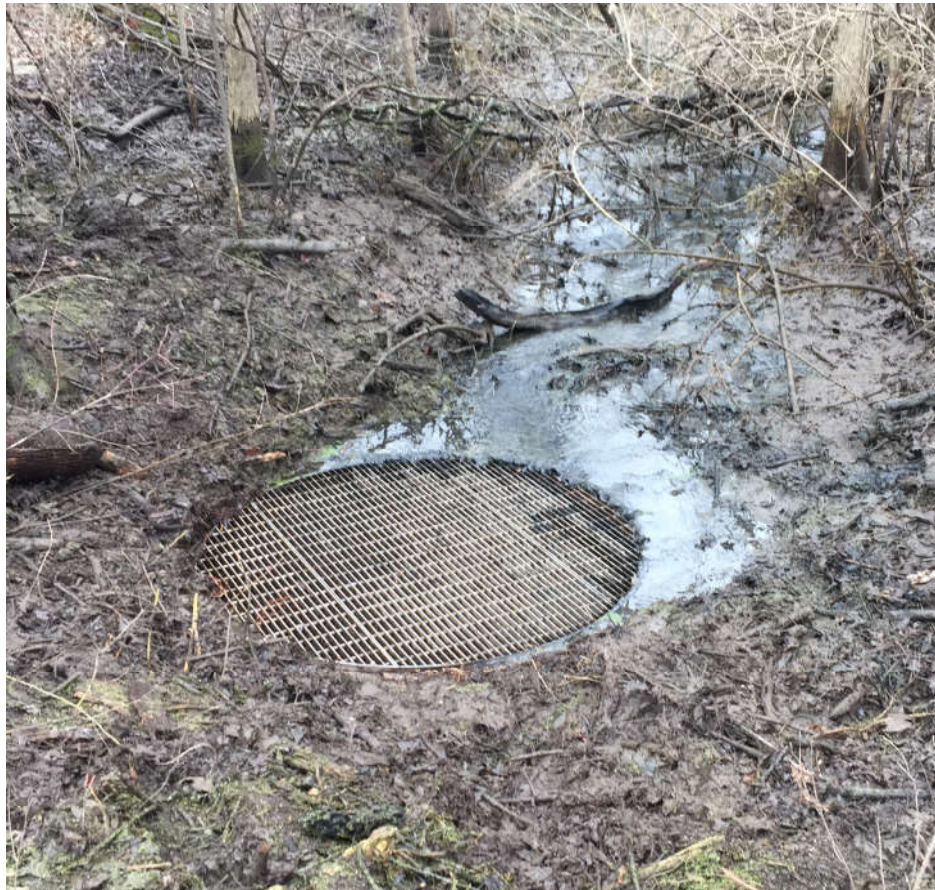
Hills N' Dales Culvert Inlet after removal of leaves/debris
