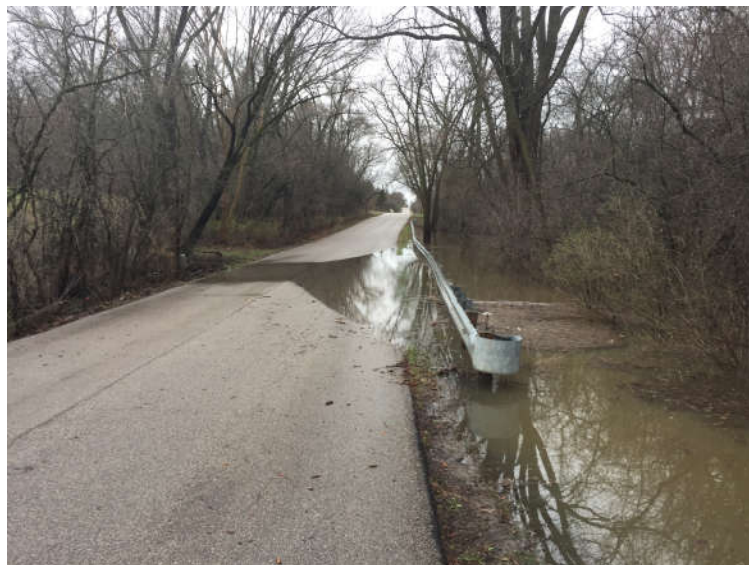
Dundee Lane Culvert- Overtopping after April 2017 Storm Event
