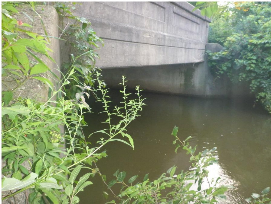
Figure 2. Bridge elevation looking southwest.
