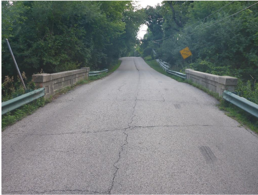
Figure 1. Porter Bridge looking west.
