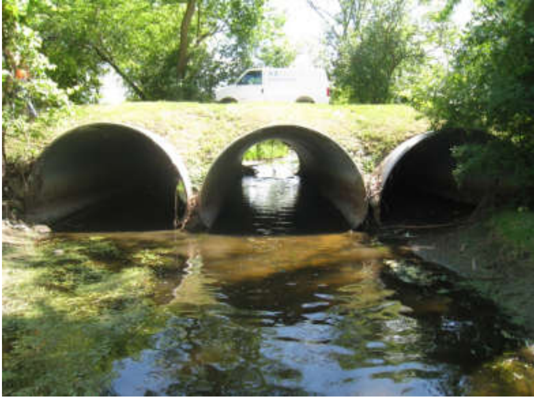
Spring Creek Culverts (Spring Creek Road, construction date unknown)
