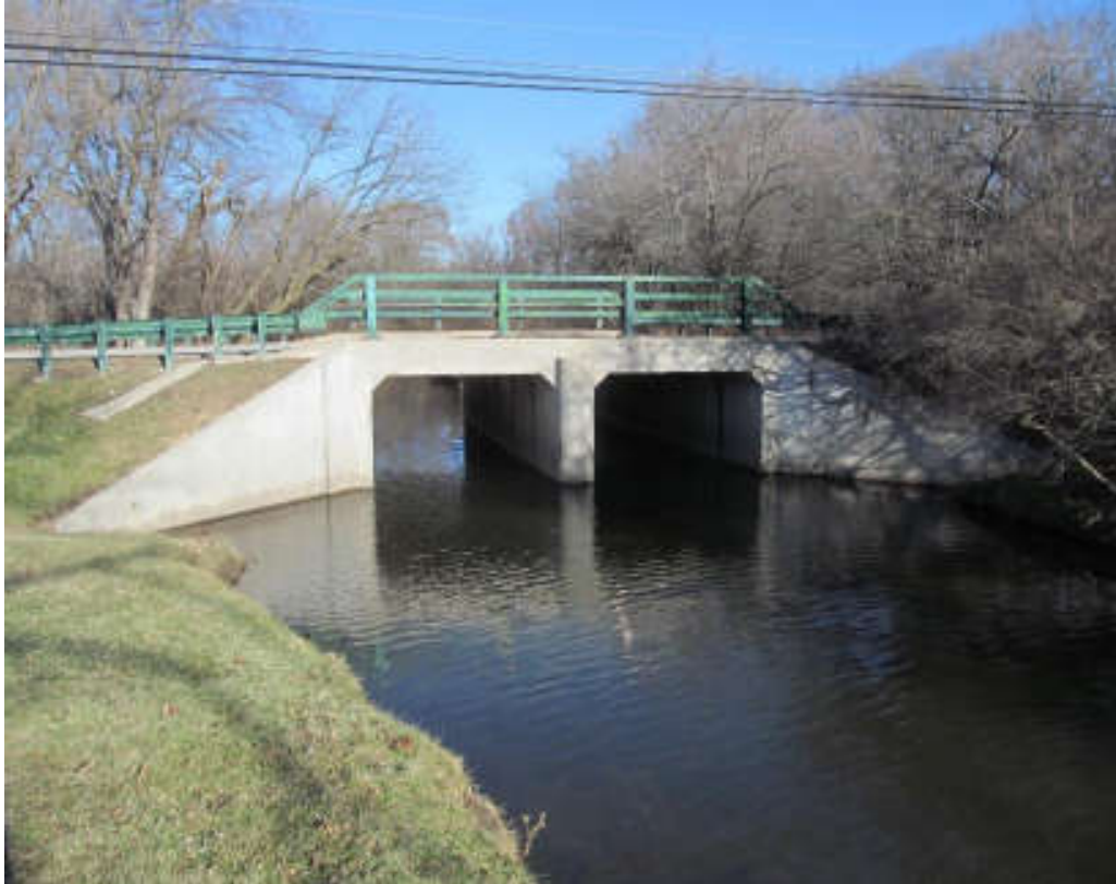
Green Rail Bridge (Oak Knoll Road, constructed in 1988)
