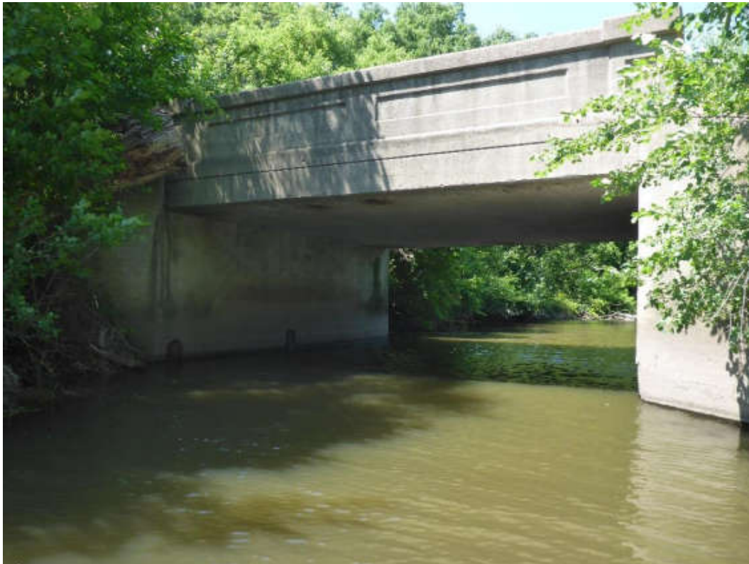
Porter Bridge (Oak Knoll Road, constructed 1926)
