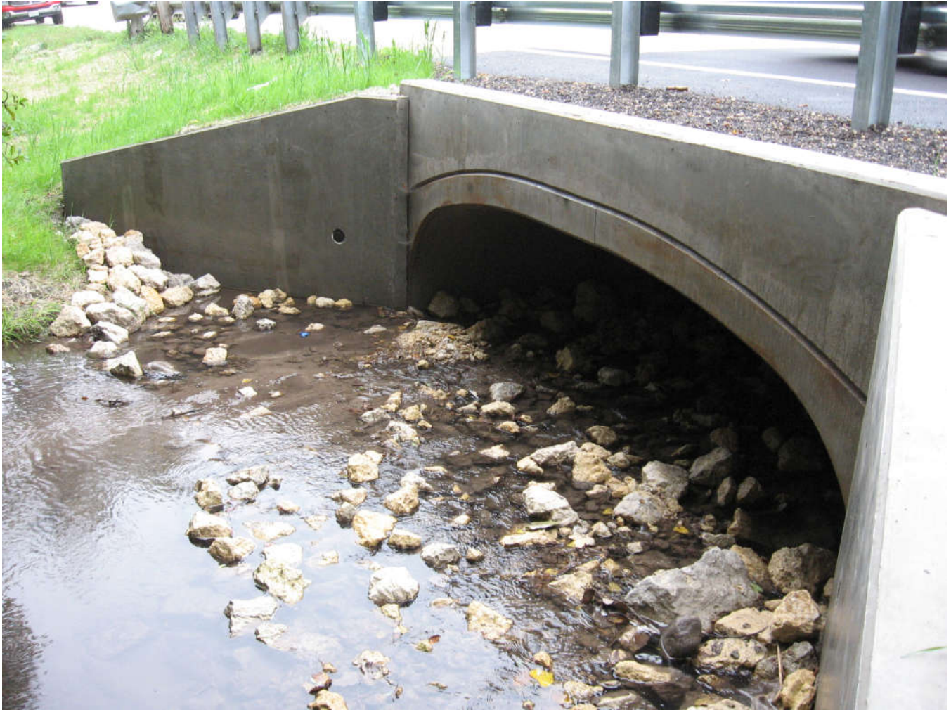
Algonquin Road Culvert (Constructed 2008)
