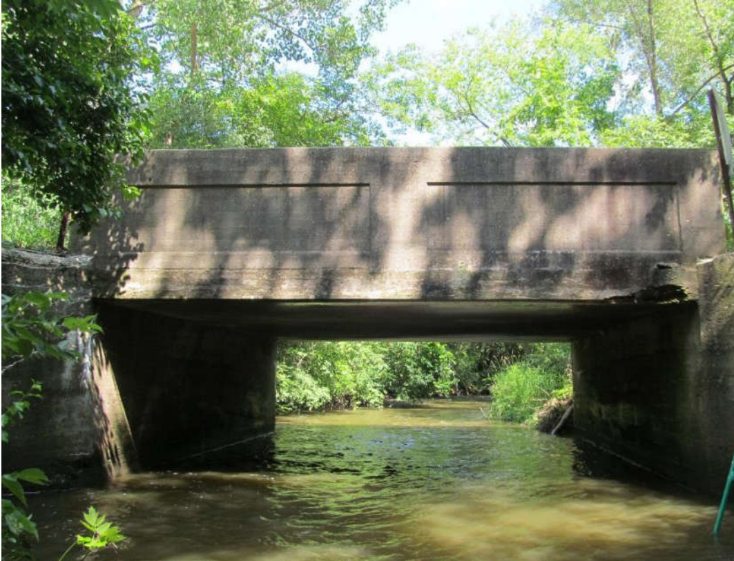
Old Hart Road Bridge (Constructed c. 1920, repaired in 2015)
