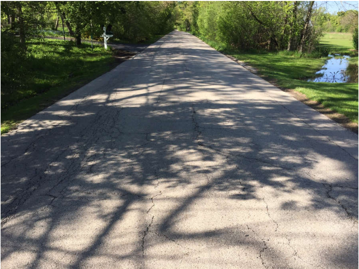
Fig. 6 – Old Hart Road- North at Existing Culvert to be Bypassed
