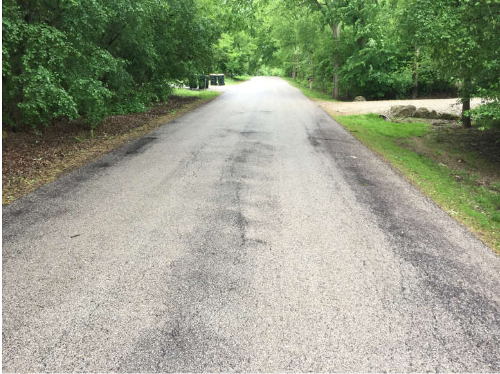
Fig. 14 – Merri Oaks Road- West of Veterans' Crossing, looking west
