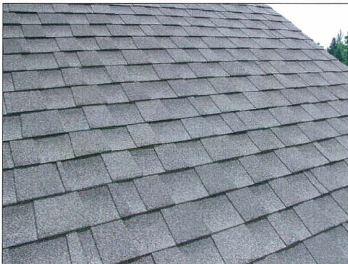
6. OVERVIEW OF LEAK AREA
