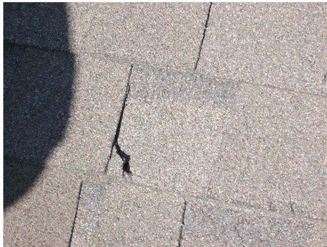
9. CRACKED SHINGLES
