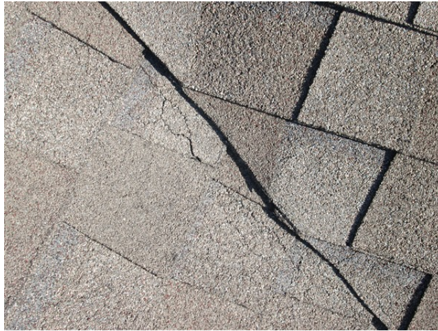
7. CRACKED SHINGLES IN VALLEY
