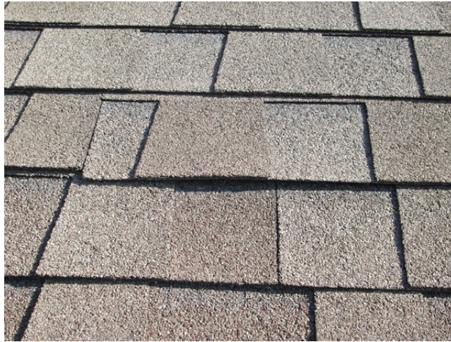
10. BACKED OUT FASTENER
