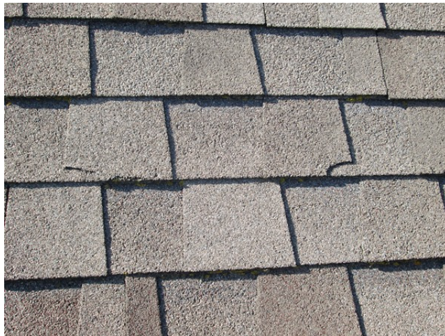
11. DAMAGED SHINGLES
