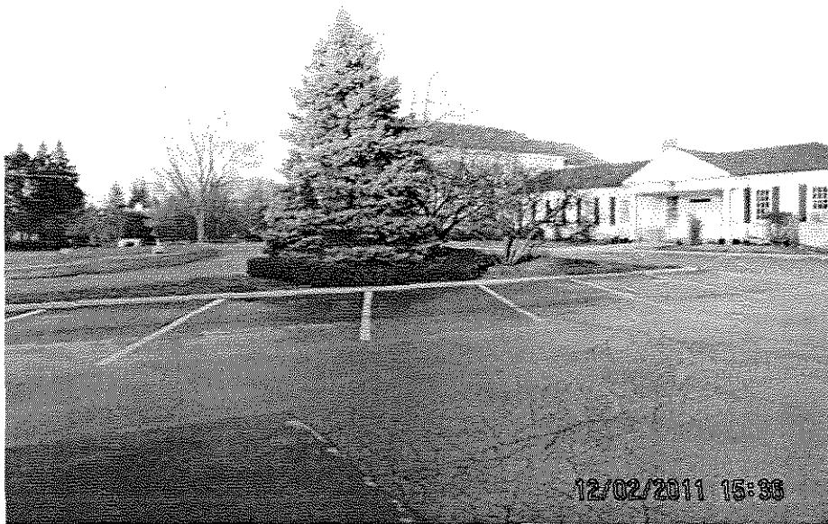
Comment: Photo of the church facing northeast in the parking lot.
