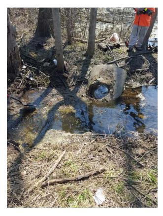
The remaining pipe that drained stormwater from the structure in the photo is a clay pipe that will be considered for replacement as part of the 2016 Road Program.
