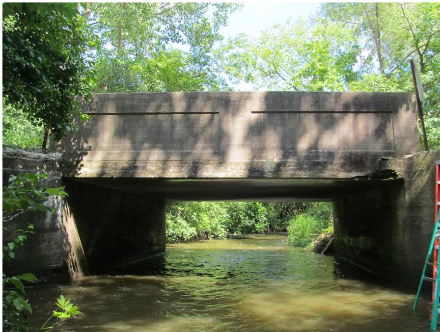
Figure 2. Bridge elevation looking east.
