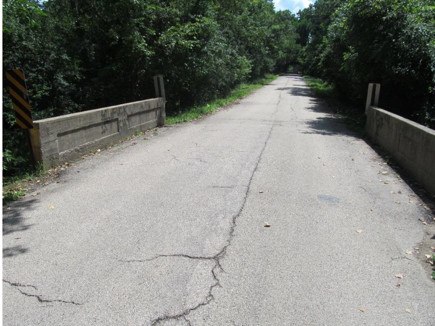
Figure 1. View of Old Hart Road Bridge over Flint Creek looking south.
