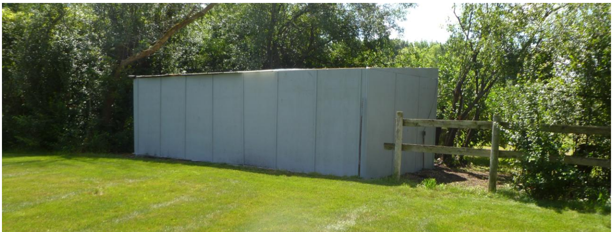
Photo taken 08/13/2015 after construction
